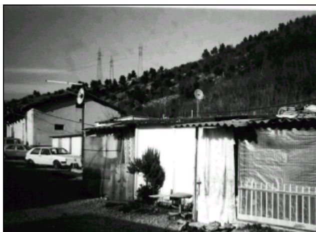
Collective Centre barracks
