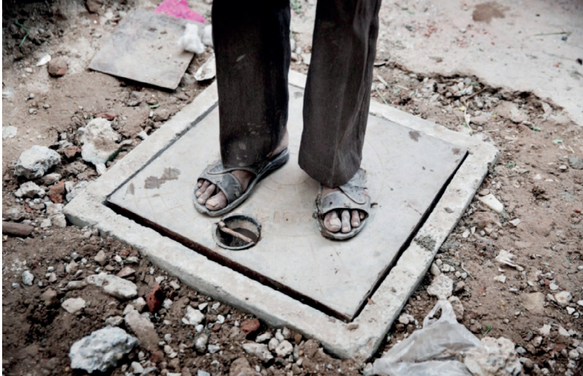
Figure 5. One new sewer chamber (photograph: Adam Ferguson, WaterAid)
