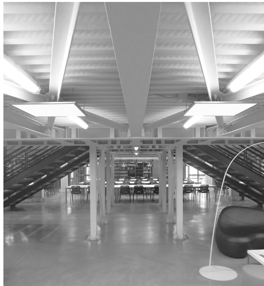
The “Cultural Flow Zone” of Ca ‘Foscari at Zattere - view of the reading room inside “tesa n.1” and of the historical wooden beams that are integrated with the modern steel structure of the mezzanine
