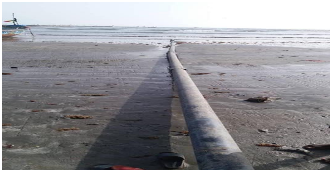
Figure A5. Waste Discharge Pipe from the Golden Lead Fishmeal Factory into the Sea.
