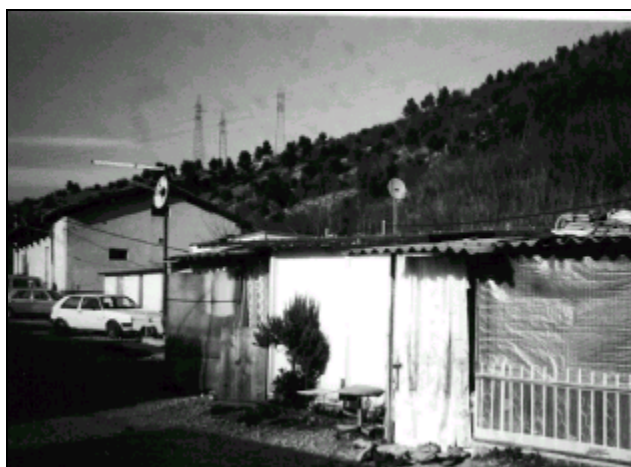
Collective Centre barracks
